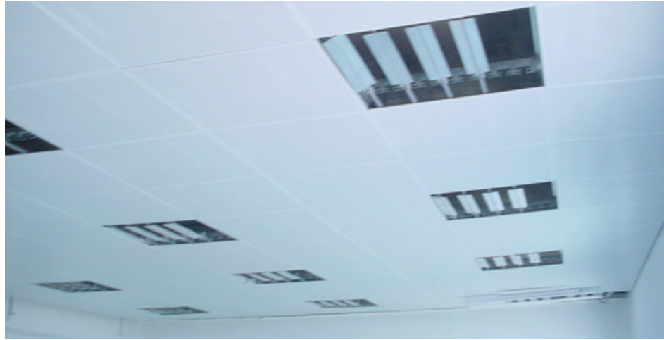
Figure (3.5): Ceiling panel
