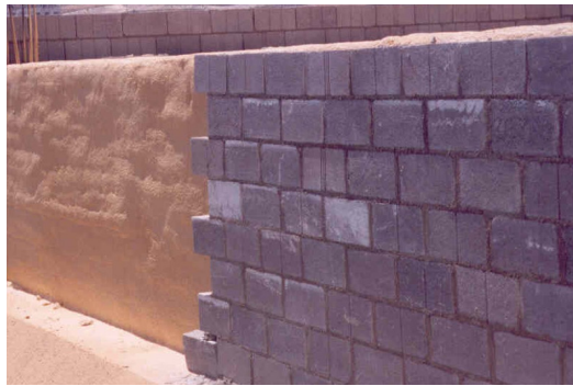
Figure (3.2): Sprayed polyurethane
